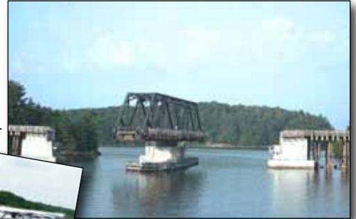
The Parry Sound Swing Bridge
